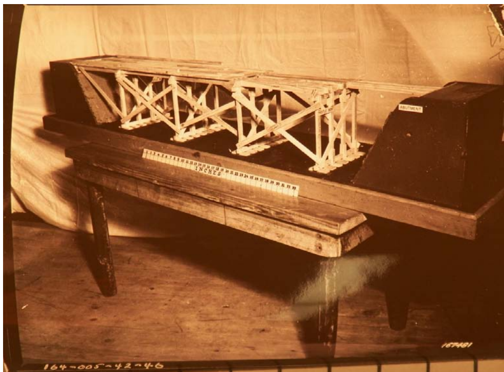
SC 157481: Model of dressed timber bridge (1 inch = 3 feet) H-15 loading. Constructed as training aids for teaching men theory and methods of bridge design and construction. 12/29/42 Photographer T/4 Edgar S Bagley
