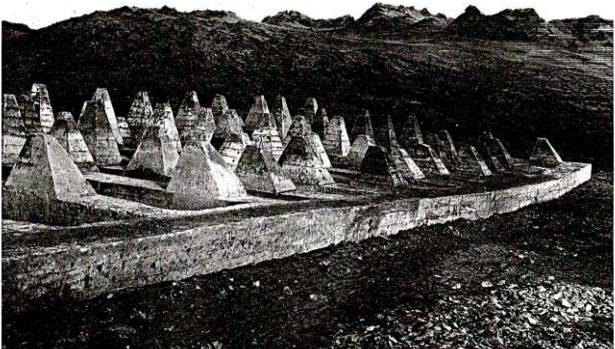
Figure 159: USATC, Area B, Practice Assault Beach, dragon's teeth anti-tank obstacles (U.S. Army, courtesy of Richard Bass)
