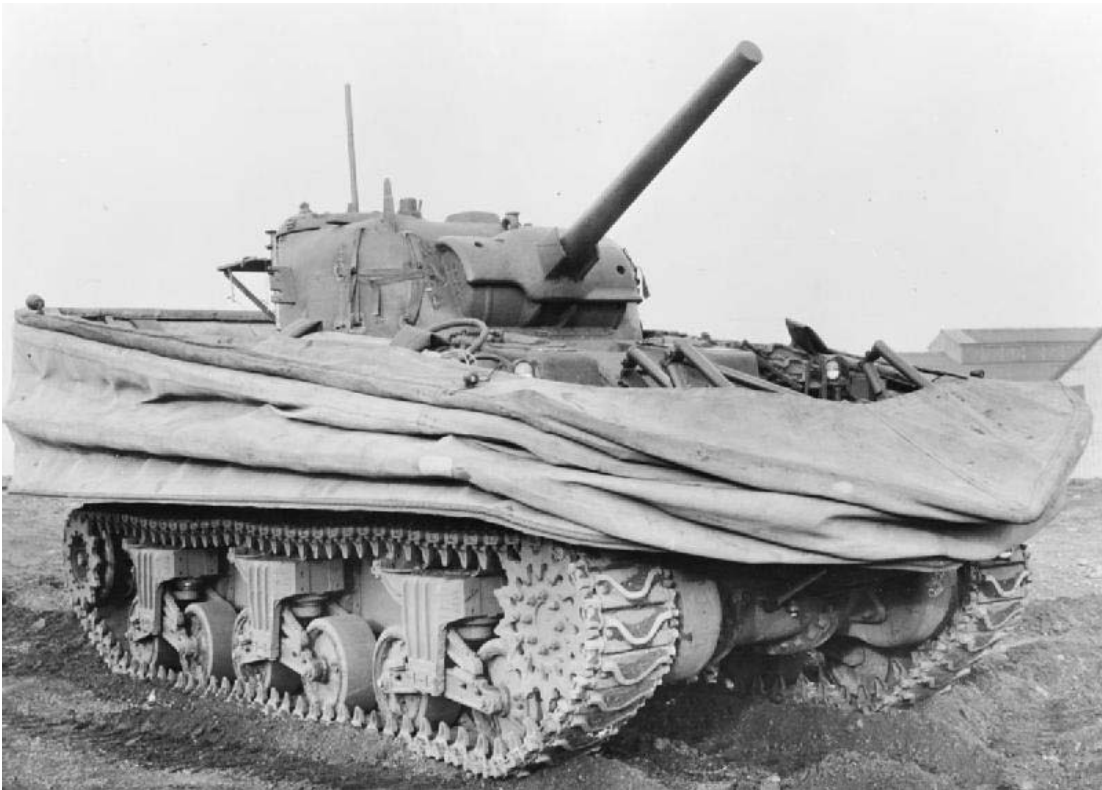
Figure 253: Duplex Drive (DD) Tank, Variant of M4 Sherman medium tank used by 743 rd Tank Battalion (United Kingdom)
