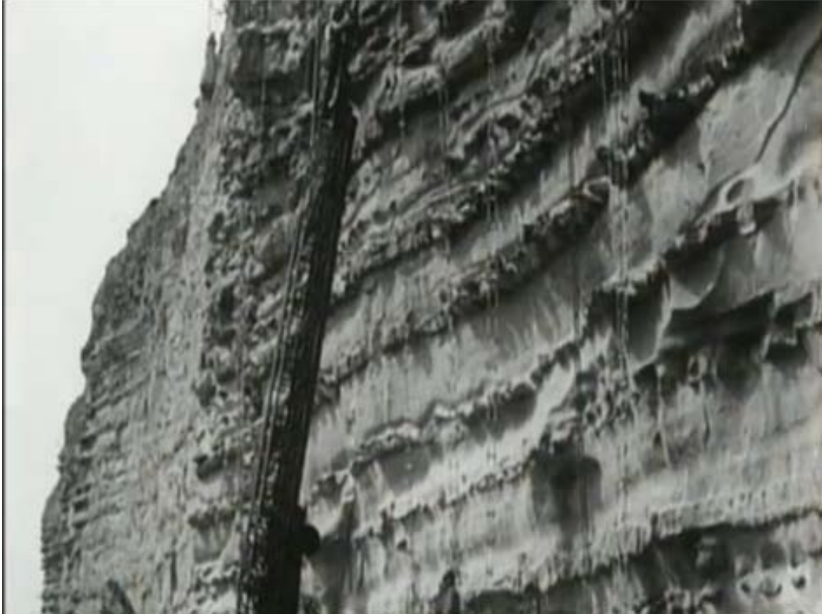
Figure 211: London fire-brigade ladders extended up cliff at Burton Bradstock (IWM)
